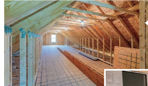
Habitable 12/12 with 3/4 deck and 2x6 endwalls. R30 insulation under floor
