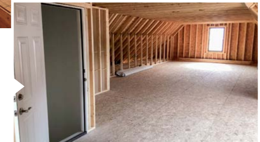
Habitable 12/12 with 3/4 deck and 2x6 endwalls. R30 insulation under floor
