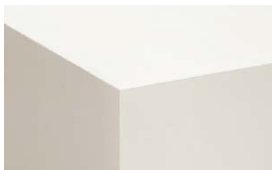
Finished Ceiling Joint
